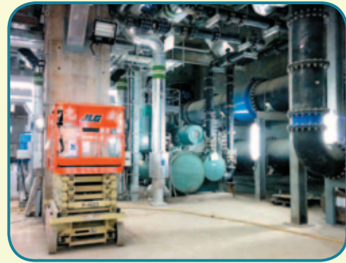
南廠制冷機組 South Plant Chillers
